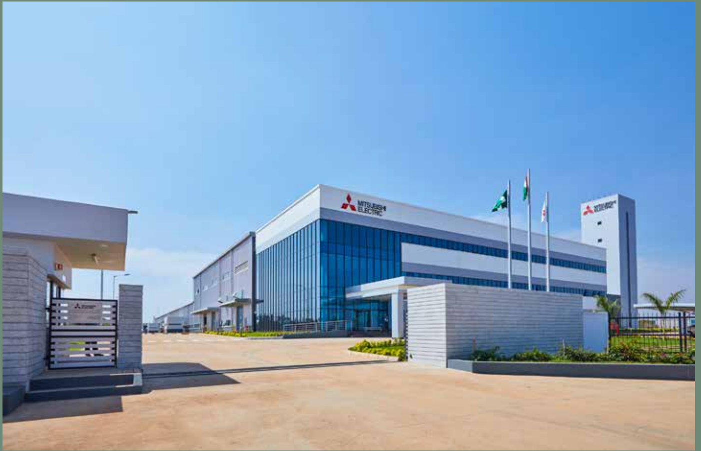
Mitsubishi Elevator India manufacturing facility in the Vemagal Industrial Area of Karnataka state
