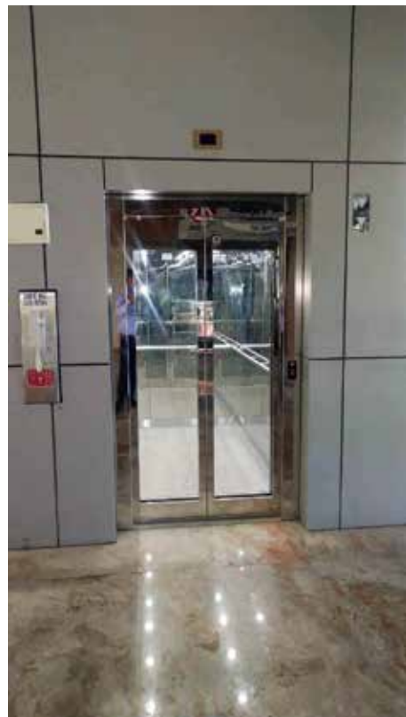
JLPL installed two 20-passenger-capacity lifts at the terminal.
