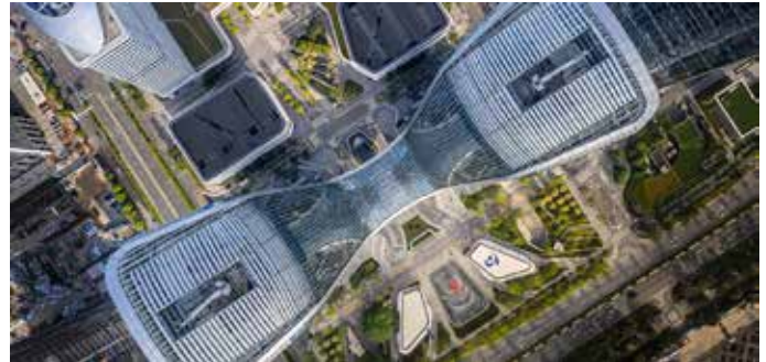
The One Excellence development in Shenzhen, China; image courtesy of World Architecture News
