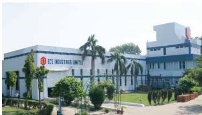
The ECE manufacturing facility in Ghaziabad
