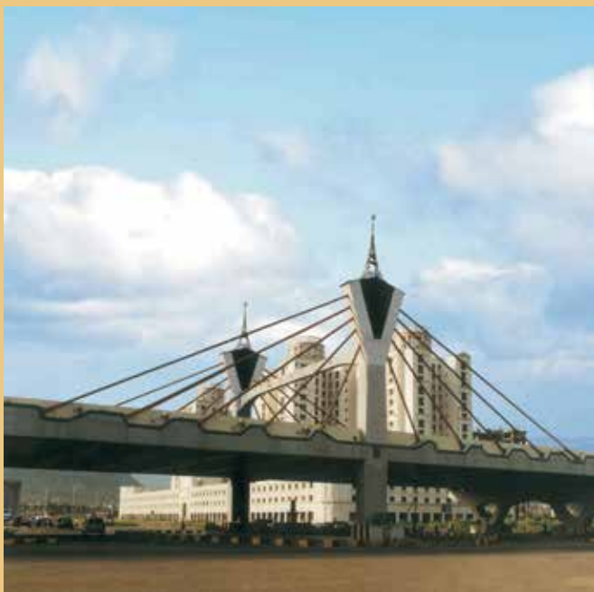
Kharghar Bridge; image courtesy of CIDCO
