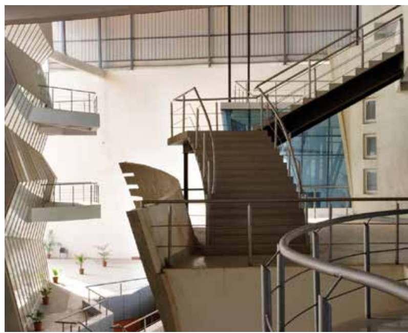
The multilevel building's numerous staircases show off the structure's modern flair. In addition to its elevators, the campus has a chairlift to provide accessibility.
