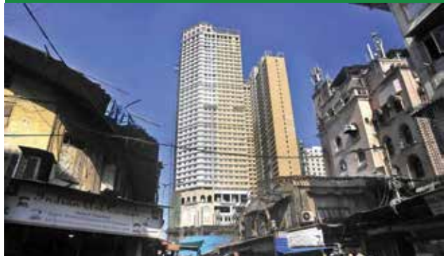
Residents have moved into the new towers; photo by Emmanuel Yogini.
