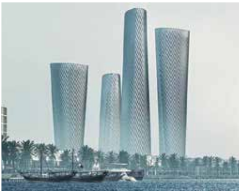
Planned project in Lusail City Financial District, Qatar; image courtesy of HECC
